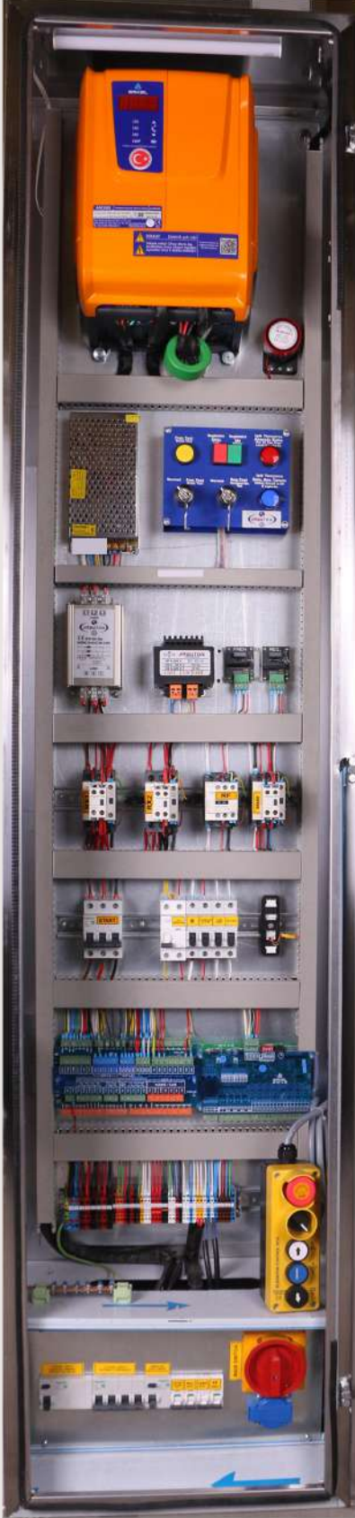
mrl dislisiz kontrol panosu (mrl gearless control board)
